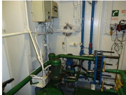
Detroit engine room (Schottel water jet engine) cooling systems for schottel and aircon systems.
